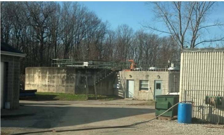
The Sewer Plant Must Monitor and Treat Pollutants
